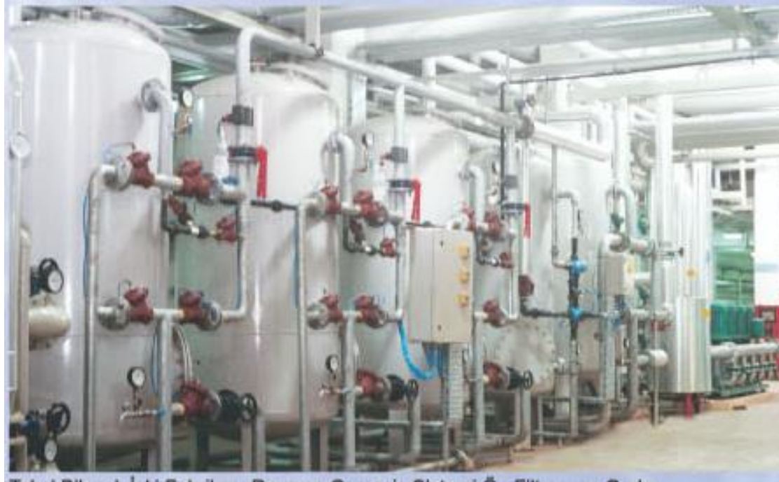
TEKEL WHISKY FACTORY (BEVERAGE) Process Water Preparation System Demineralization System 5 m 3 /hour
