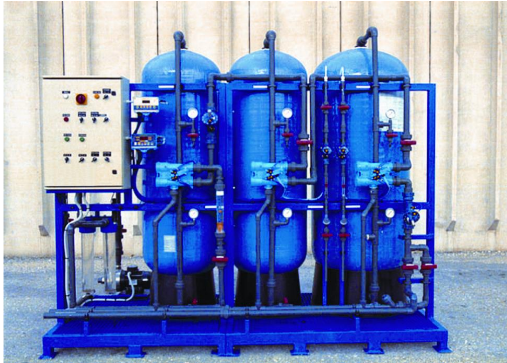
OTOKAR AUTOMOBILE INDUSTRY Process Water Preparation System Recycle Demineralization System 5 m 3 /day
