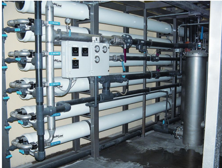
BIRLIK ENERGY ELECTRIC PRODUCTION OTOPRODUCTOR GROUP Boiler Feeding and Cooling Water Preparation System Reverse Osmosis System with Prefiltration Group 33 m 3 /hour
